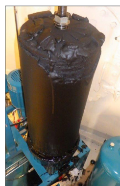
Dirty CJC® Filter Insert, having removed the contaminants from the fuel.
